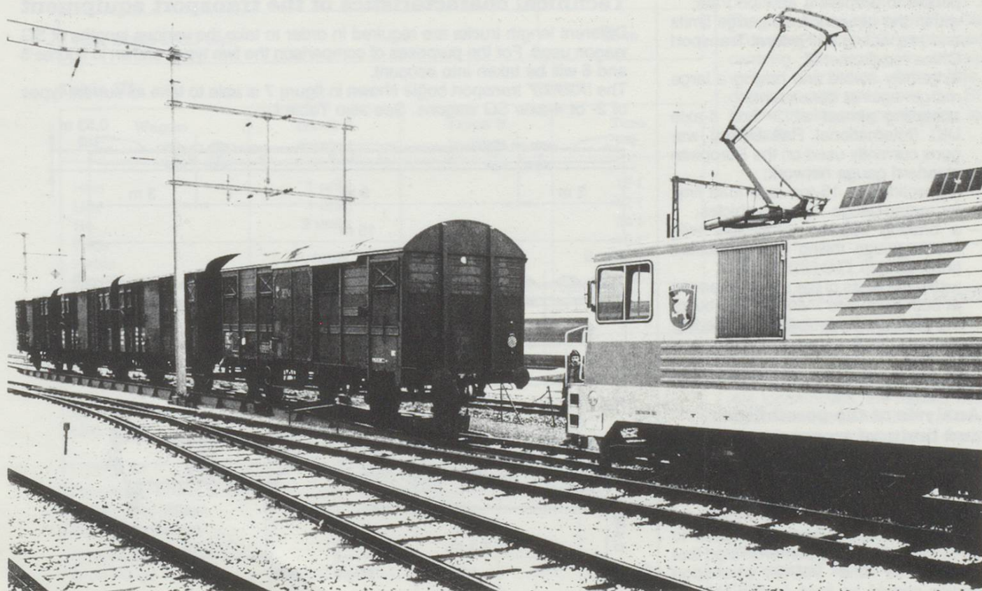
Fig. 2. The transfer station at Palézieux.
