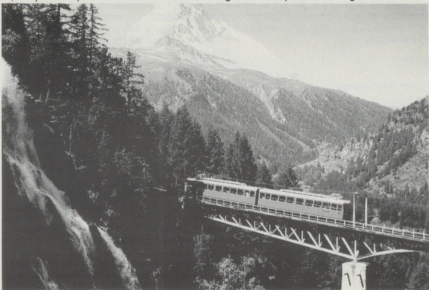
Bhe4/8 crossing the famous Findelenbach bridge.
