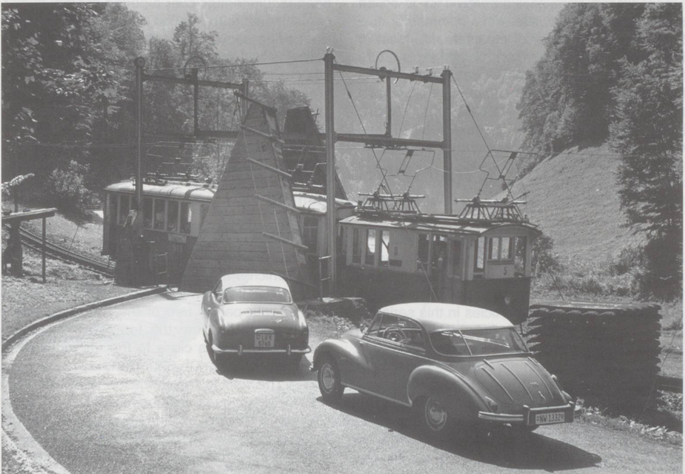
Grünenwald: 1961. An HGe2/2 No.5 [built 1913 by SLM/BBC] of the Stans Engelbergbahn passes the Bascule bridge. Photo: [LSE] Hardy-Randall collection
