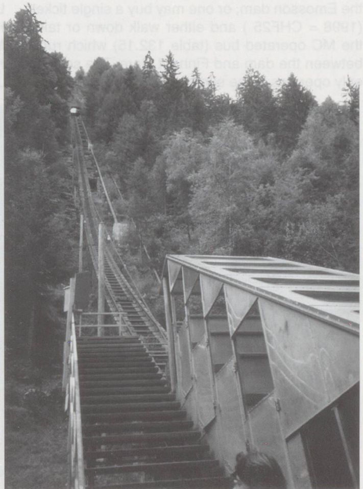
Le Châtelard: Lower Funicular showing the haulage rope lifted well off the guides. Photo: Anne Williams
