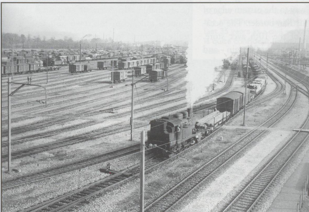
Muttenz. SBB Loco E4/4 (converted C4/5) on marshalling duties
