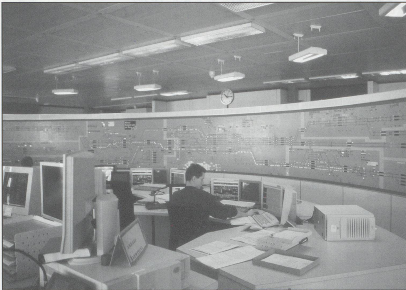
Olten Control Centre mains panel. The ETCS section is worked on a separate VDU (IECC) type panel.
