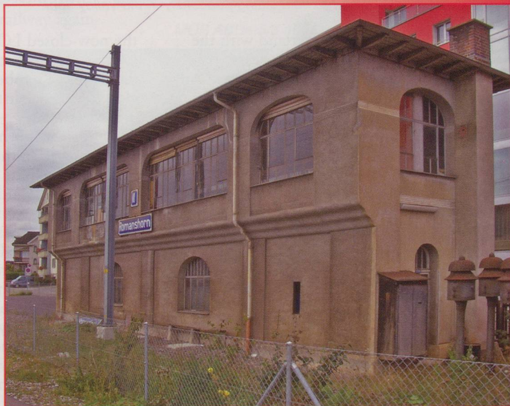
Romanshorn II signal box. It is hoped to incorporate this building in the future 'Locorama' museum.
