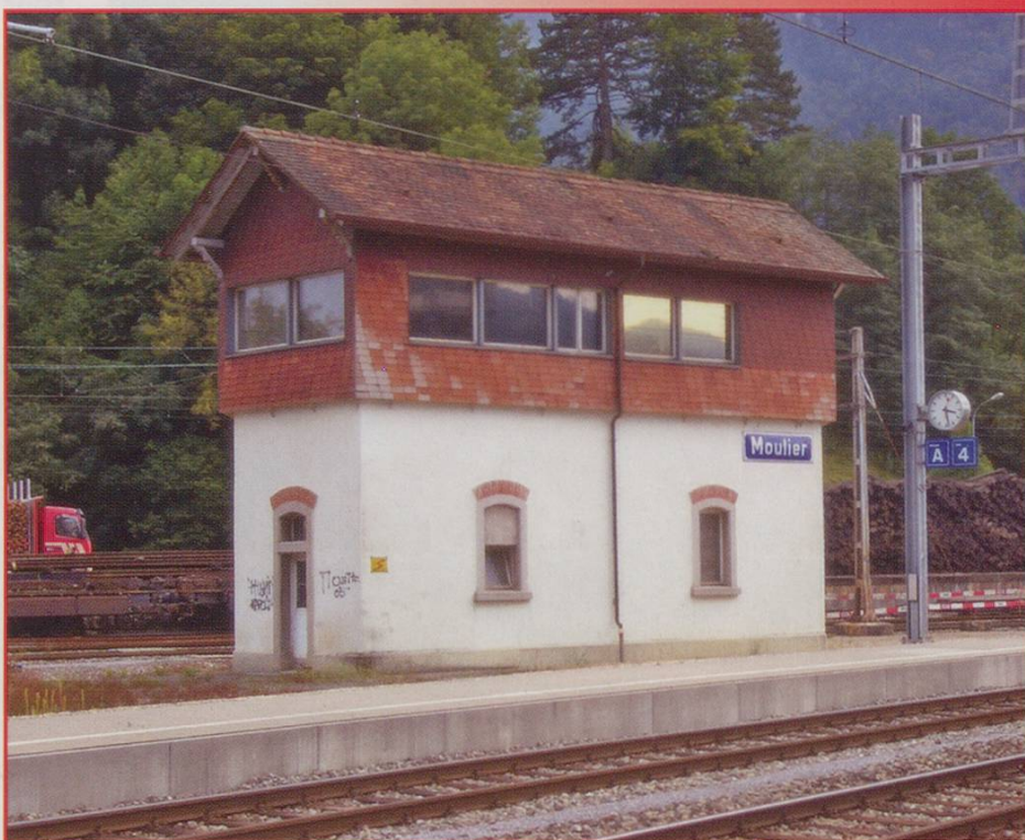
Moutier. There are two signal boxes at this location. This is the north box, where the lines to Basel and Solothurn diverge.
