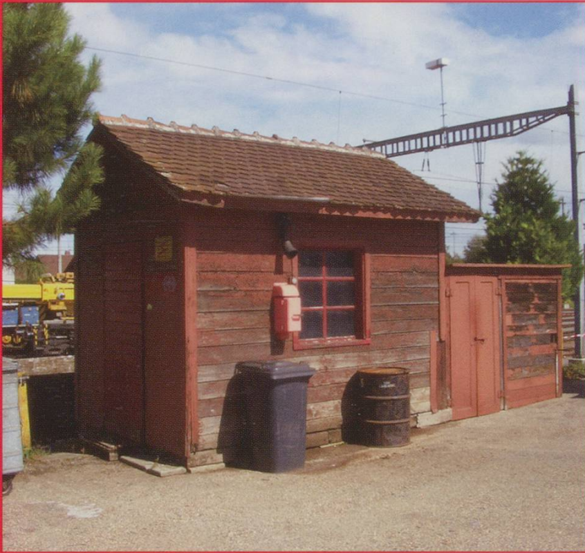
Regional examples of railway huts:
