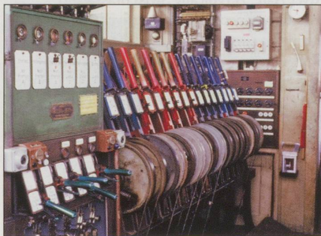
BOTTOM: Frenkendorf station: Bruchsal lever frame, with Hasler route and block instruments, as they were in almost every station. Sometimes they even stood in the open.
