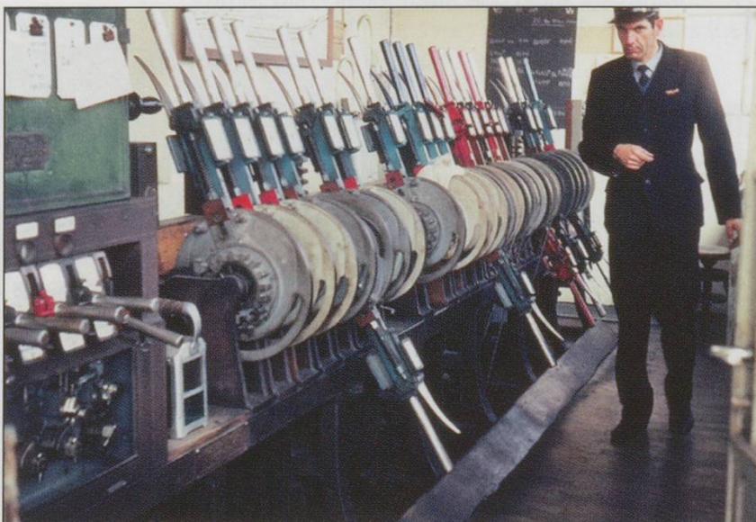
BOTTOM: 'Bruchsal' lever frame, at Cossonay station, 17/10/1968.
