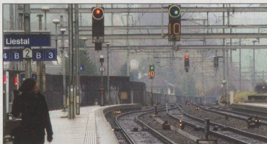
BELOW: Signals at Liestal. Platform 3 signal at stop, the through track clear to enter the section at 100 km. Note also the dwarf signals on the main lines.
