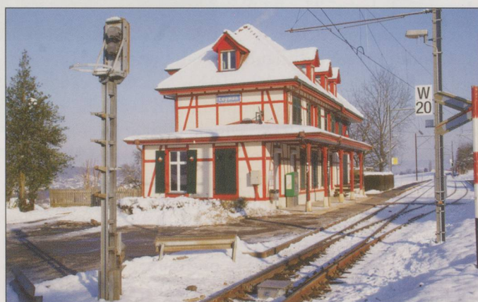
TOP: Leymen Station and Custom House. The freight customs shed was accessed from Switzerland by the double doors and exited to France at the other side of the building.
