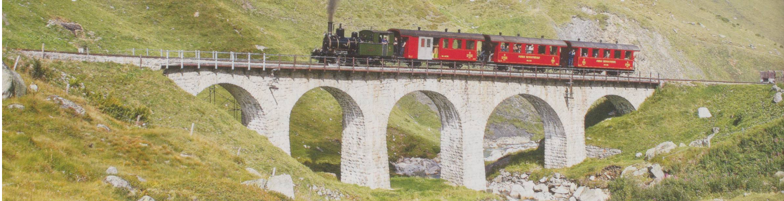
The magnificent scenery of the DFB line at the Steinstafel Viaduct.
