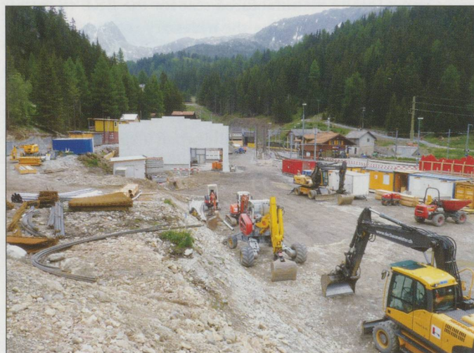
Albula Tunnel Works.
