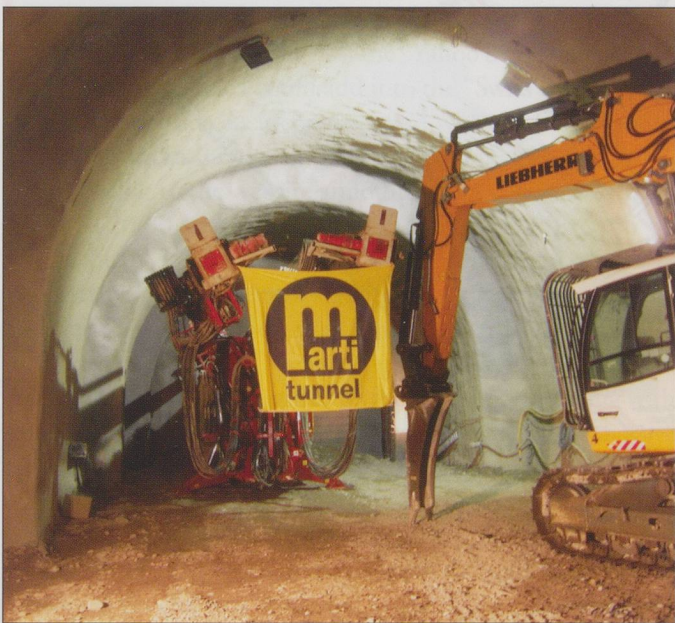
Digging the Champel tunnel. (26.9.2015)
