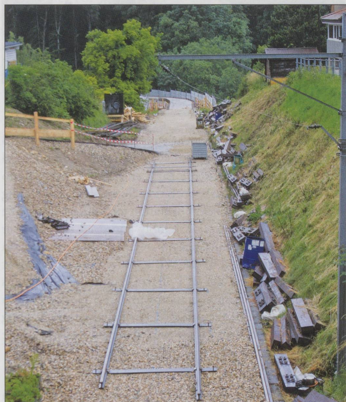
Nyon St Cergue temporary closure, changing from bus to train and laying new track. Photo: Gordon Wiseman
