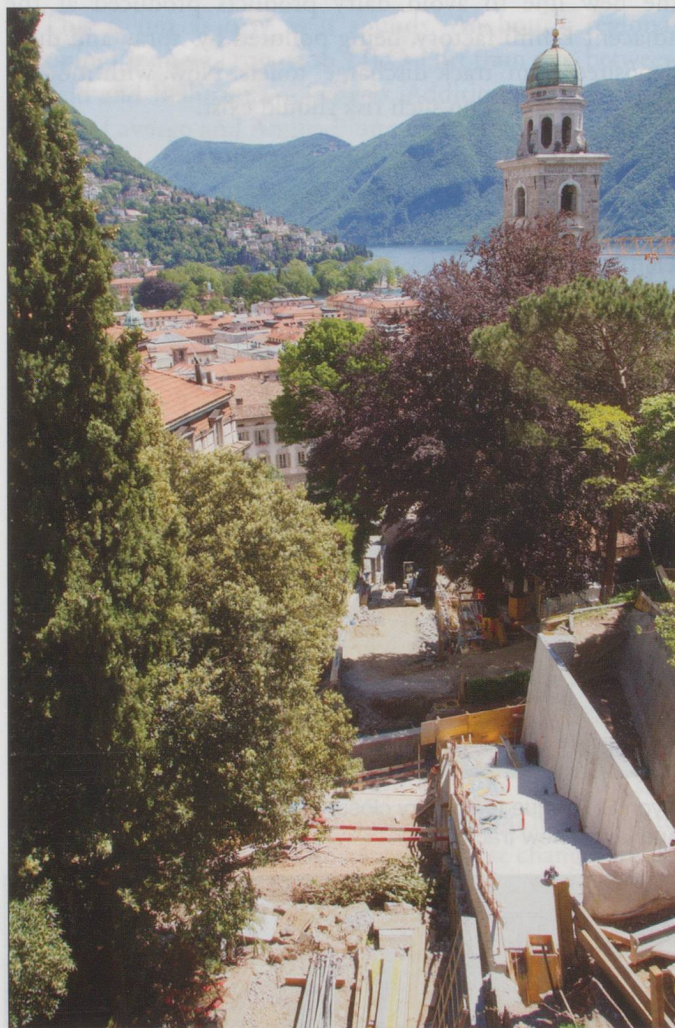
A view over Lugano with work in progress on the funicular.
