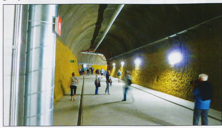
ABOVE: 460 006 08 and the dedicated rake. LEFT: The evacuation tunnel. Photos: Trevor Gauntlett
