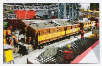
former habitat. The large, impressive works sites, for example the one at Preda with its exhibition, will disappear all togetheronce work is complete. Spoil from the excavation has become a raw material, being used as much as possible on site to supply aggregates for concrete, with the excess being sold-on commercially.
