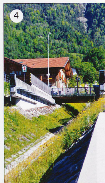
4. This gives a better idea of just how steep the waterway is, and how much extra space for water and debris is achieved by moving the bridge. The controls for the bridge are also in the picture.
