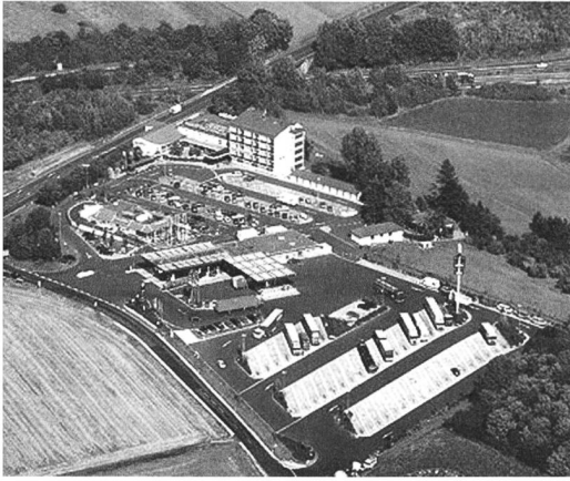
Multi-functional service area, Baden-Württemberg/Germany, 1996, photo.
