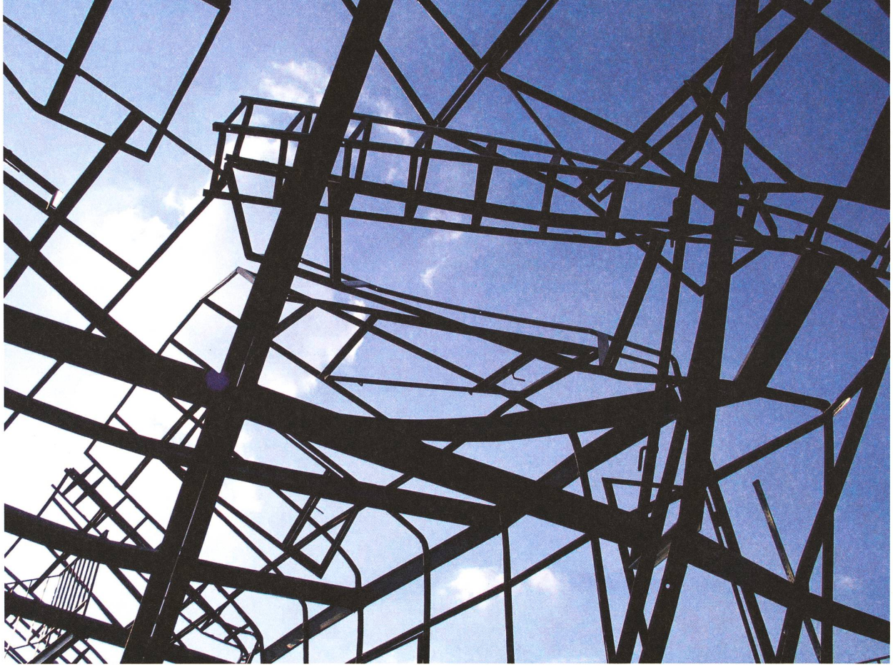
fig. a Monika Sosnowska, '1:1', 2007, open air production and deformation of the construction in Warsaw.
