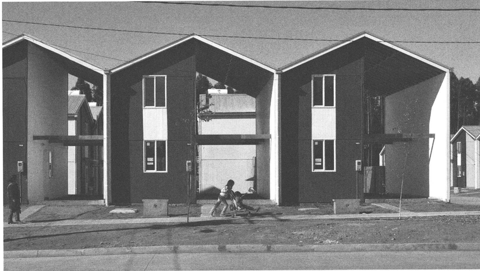
Villa Verde Housing, September 18 th 2013, Constitución, Chile © ELEMENTAL
