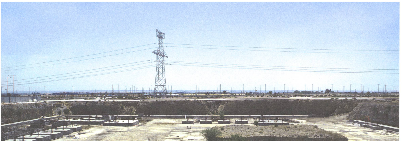
Interrupted foundations, PAU El Quiñón, Seseña, Toledo. Photography: Isabel Concheiro, 2014.
