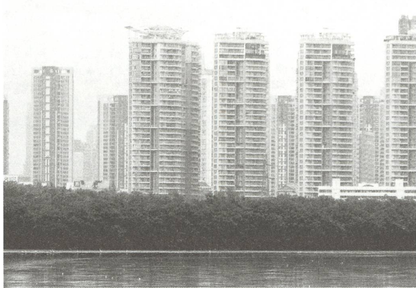
Gated community under construction, Qianhai area, Shenzhen. Photography: Ting Chen, 2014.
