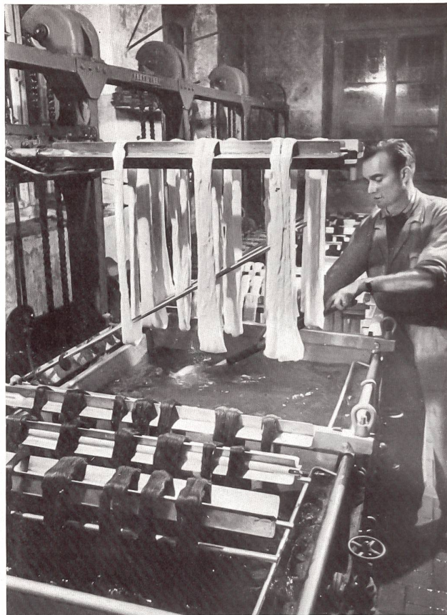
Hank dyeing machine for silk twists.
