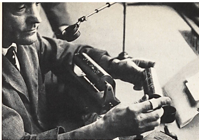
Engraving prior to roller printing. (Cilander A.G., Herisau)
