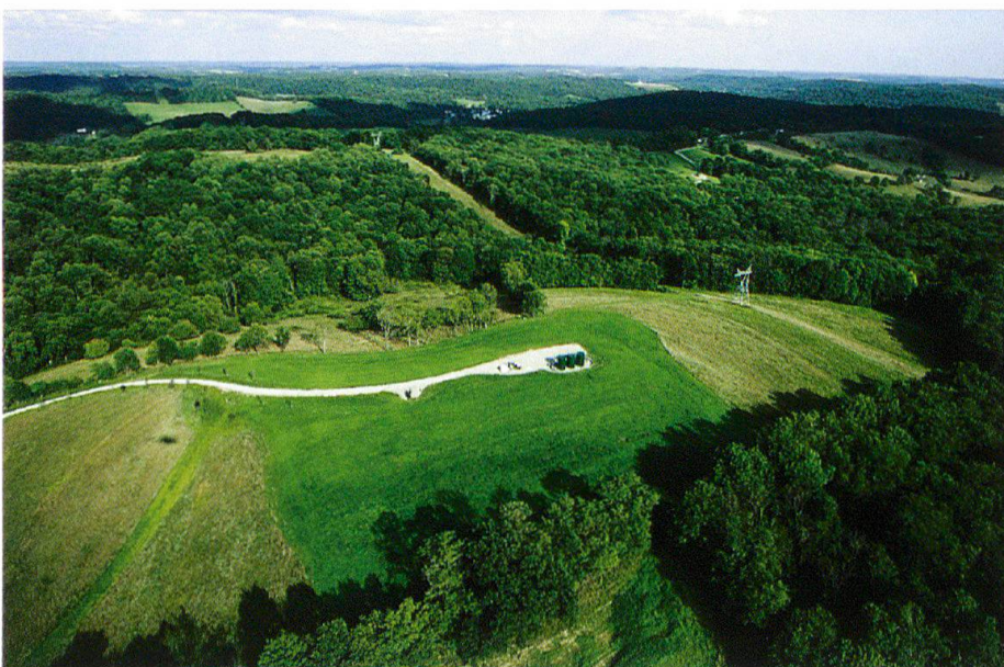
Fig. 4: Shale gas multi well production site Range Resources (Pennsylvania). Dark green area around production site indicates the surface previously used during drilling and stimulation.
