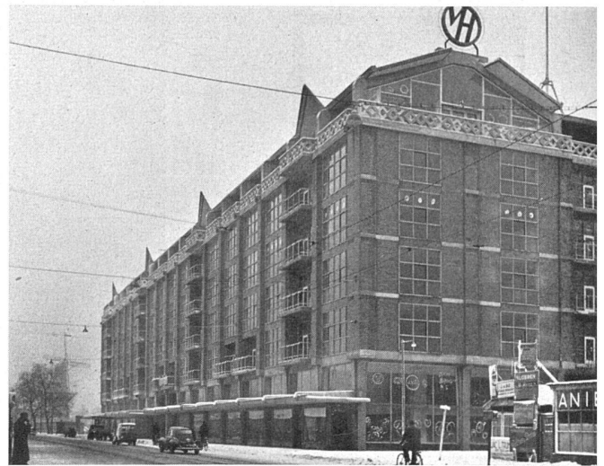
Mietfabrik Goudse Singel. Ladenfront | Usine locative (II), vue générale | General view of flatted factory (II)
