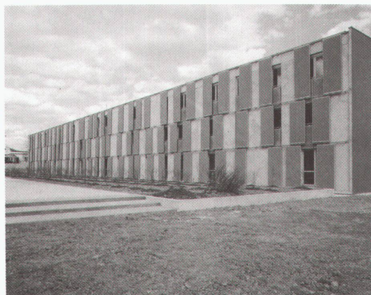
■ Graz-Strassgang residential building, 1994. The building has a minimal base, little more than a keyed joint over the floor slab on the ground floor. All the apartments have an equal amount of external space and are equipped with French windows. The garden area is "no-man's land".
