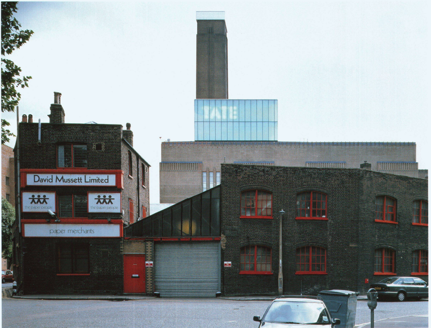
Tate Modern, 1994–2000 Architects: Herzog & de Meuron, Basel Jacques Herzog, Pierre de Meuron, Harry Guggler, Christine Binswanger Project architect: Michael Casey Associate architects: Sheppard Robson + Partners, London Interior design: HdM with Jasper Morrison Engineers: Ove Arup Partner, London Landscape design: HdM with Kienast Vogt + Partner, Zürich
