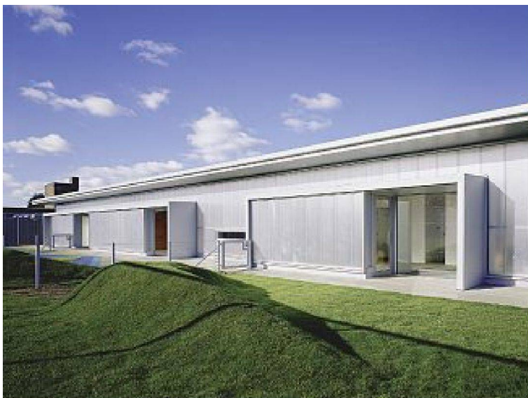
John Perry Children's Centre, Dagenham, 2006. – Bild: H el ene Binet
