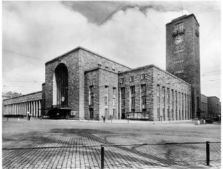
Hauptbahnhof in Stuttgart, 1911–27
