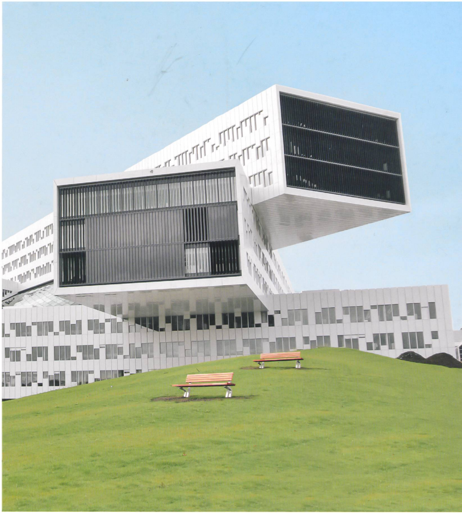
Statoil Headquarters, Oslo
