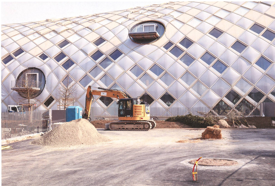
Omega-Neubau (Shigeru Ban)
