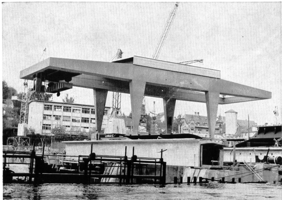
120 t Portalkran KW Schaffhausen
