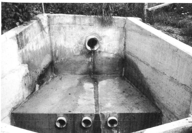
Reference number 2.200(2). Seepage measurement at the downstream toe of an embankment dam. The seepage water is measured by calibrated container at the outlets which drain a different sector of the dam each.
