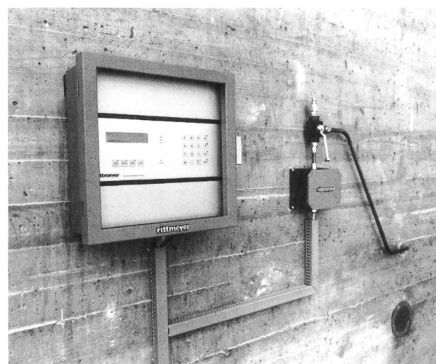
Reference number 1.000-1(2). Quartz sensor (replacing the pressure balance) for determining the reservoir level by measuring the hydrostatic pressure.
