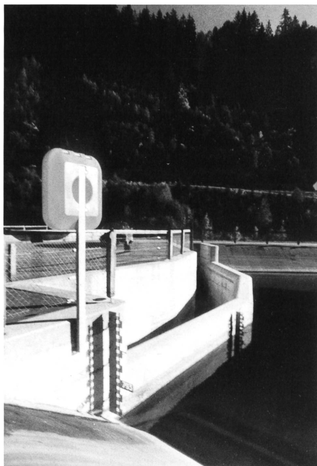
Reference number 1.000-3. Staff gauge. Calibrated metal scale to determine reservoir water level.
