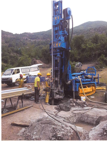
Figure 3. Drilling works for inclinometers with sub-contractors Altea Geostudio2000 at Porava.
