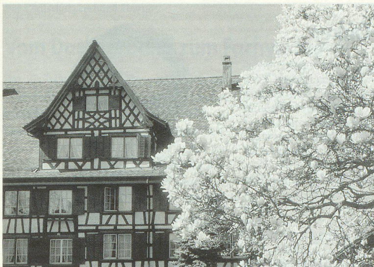
Riegelhaus in Roggwil.
