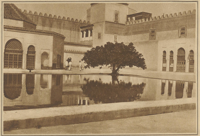
Innes des Sultanpalastes in Marakech
